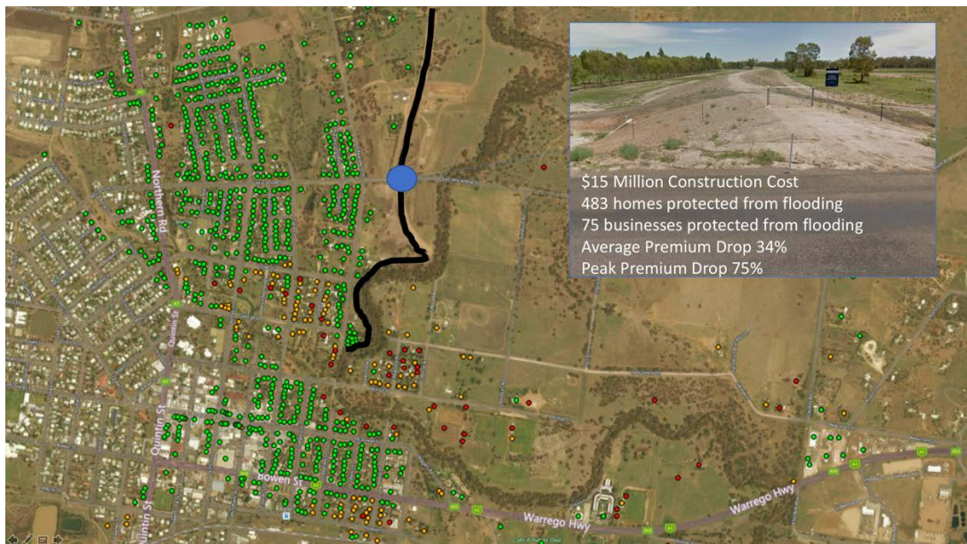
Figure 10 – Properties in Roma QLD exposed to flooding post-mitigation
